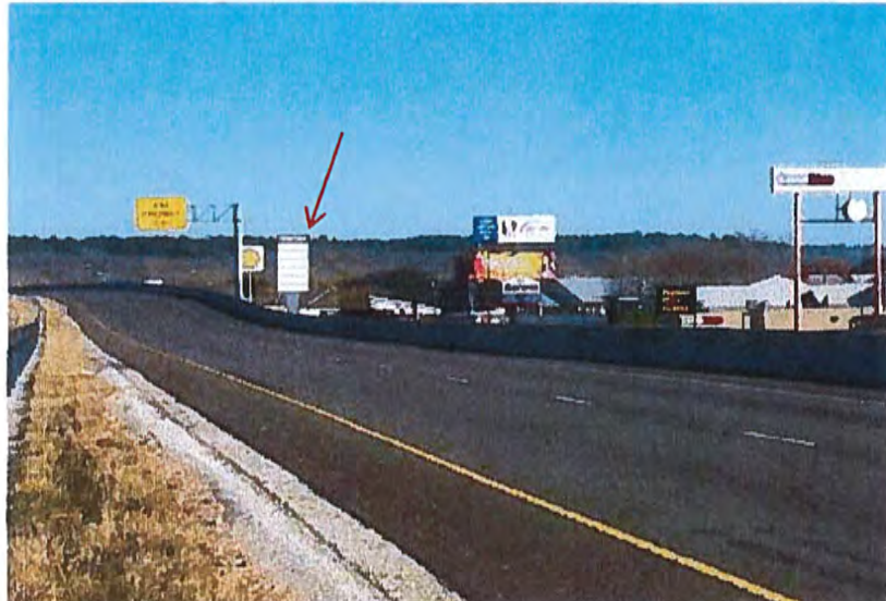
50' Sign from Highway 71 Eastbound
