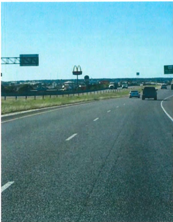
Westbound 71, South side of 71
