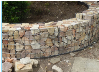
STORMWATER COLLECTION OVERFLOW BLOCKS / GABIONS
