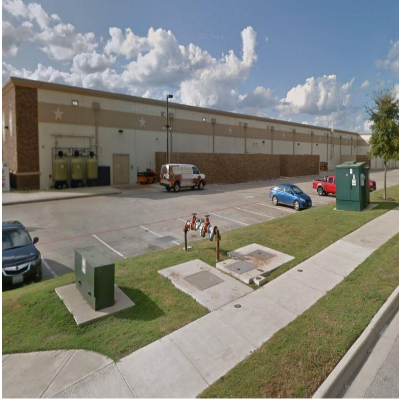
Example of 2 transformers to provide power to multiple locations on the same site (Buc-ee's)
