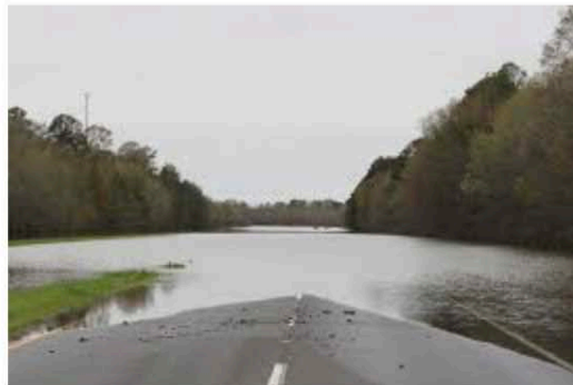
Photos: Highway 165 flooding - Bastrop ... bastropenterprise.com
